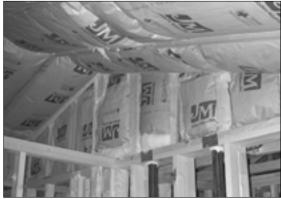
Knee walls were commonly insulated as shown in the photo on the left. Insulation batts were installed on the attic side of the framing, leaving a significant air space between insulation and wallboard. Attic air could move through this gap. The photo on the right shows knee wall insulation that was effectively installed between the framing. These batts will be in substantial contact with the wallboard as required by the code.
