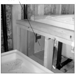
The solution is easy and inexpensive, but requires a change in construction sequence. The air barrier behind this tub was installed before the tub was set in place. This was observed in about half of the homes under construction.
