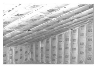
This is an example of effectively installed insulation that met code requirements. Batts filled the cavities, attained full loft, and will be in substantial contact with the wallboard.
