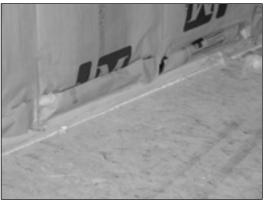
Sealing the baseplate-to-subfloor joint cut off a significant air leakage path.
