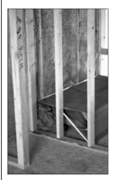
This bathtub had more than enough insulation at the exterior wall. But there was no air barrier to stop air from the outside wall from flowing through the insulation and circulating beneath the tub. From there, connections through partition walls and holes around the plumbing connected this leak to the rest of the house.
