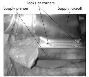
This joint between a takeoff fitting and a plenum is an example of small supply duct leaks. Some takeoffs were much leakier.
