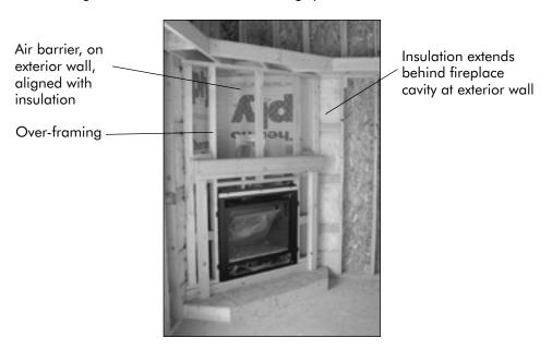
In this example, the insulation and air barrier, aligned at the exterior wall, were installed before over-framing was built and before the fireplace unit was installed. This approach will stop drafts and help the insulation perform effectively.
