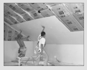
Wallboard represents the separation between the finish materials and the components and systems that determine how the house performs.
