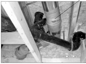
The left photo shows the typical duct sealing approach: cloth duct tape on round branch supply duct joints, nothing on other supply duct joints or return ductwork. In the right photo, duct mastic was used as a sealant. It is designed for strong adhesion and durability in this application and should last the life of the ductwork.
