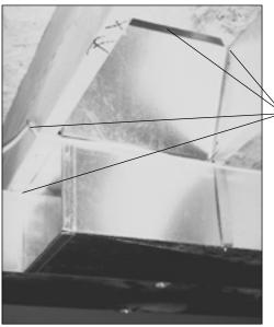
Typical leakage locations in return ductwork
