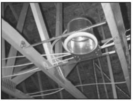
"Airtight" cans for recessed lighting reduced air leakage through insulated ceilings.
