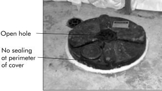
When air is drawn through an unsealed sump cover, it might bring with it radon, other soil gases or moisture.
