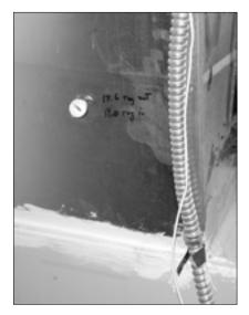
The only way to know whether a furnace is operating within the manufacturer-specified heat rise range is to measure heat rise. This test requires minimal tools and time. The testing contractor saw no evidence that heat rise had been measured on study home furnaces.
