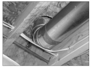
This supply duct was never connected to anything on the top end. Carpet was laid over the subfloor cutout, and the register was never installed.
