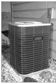
About half the study homes had central air conditioning. The compressor and condensor were located in an outdoor unit like this, with the expansion valve and evaporator coil located in the supply plenum at the furnace.
