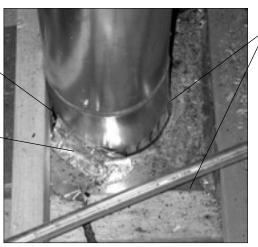
The chase surrounding this combustion air duct was partially sealed. The sheet metal collar was reasonably well done, but the rest of the job was never completed.
