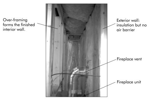
In this example, there was no air barrier at the exterior wall. This will allow outdoor air to move from the wall into the cavity around the fireplace unit and then, through cracks and holes, into the living space.
