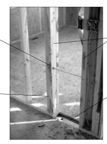
These wall studs formed two sides of a return duct. Wallboard will complete the other two sides.
