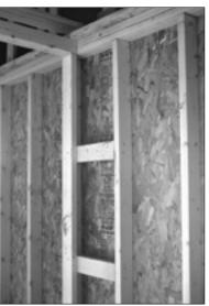
Conventional and advanced framing were used about equally at partition wall intersections in post-group homes. Conventional channel-stud framing (left) created cavities that could only be insulated from the exterior before the house was sheathed. In practice, they were rarely insulated. Ladder blocking (right), an example of advanced framing, left accessible cavities that could be insulated from the interior at the same time the rest of the wall was insulated.
