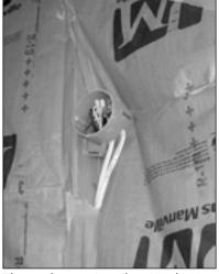
The code requires that insulation be cut to fit, without compression, around electrical and other obstructions in the insulated bay. In this case, insulation was compressed behind the box rather than cut to fit around it.
