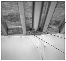
Interior view of some cantilever problems. It is not clear whether Rectangular blocking coupled with engineered "I-beam" joists left large gaps at the edges.
