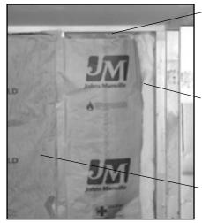
The code requires that batt insulation be cut to the correct length and installed with no voids at any edges. It also requires that the insulation must attain specified loft across the entire batt.
