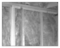
Typically-installed, unfaced fiberglass batts in a frame wall will offer reasonable performance. Note some compression of the batts in the full-width stud bays and more severe problems where a batt had to be cut to fit in a narrow cavity.
