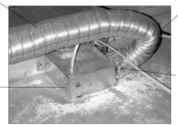
One of the few indoor air quality components installed in all study home was bath fans, intended to remove moisture and odors. In the top photo, the grille on the ceiling gave no indication about how well the fan would do its job. The attic perspective in the bottom photo illustrates some of the installation details that compromised performance.
