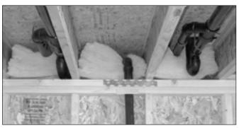
Compression of the insulation batts, voids, and the lack of contact with the subfloor above this cantilever all reduce the effective R-value of this insulation.
