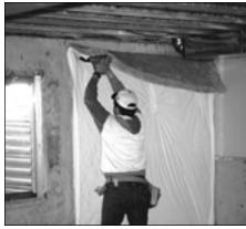
Basement wall insulation addressed one of the biggest remaining heat loss paths. The typical approach was a vinyl-faced fiberglass blanket on the interior of the concrete foundation.
