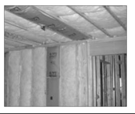
In floors over garages, R-30 batts exceeded code R-value requirements but were easier to install effectively because they were thick enough to fill the floor joist cavity completely.
