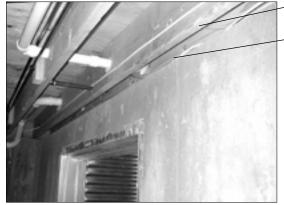
When the first floor joist was framed tight to the foundation, it left little space to insulate the rim joist. Plumbing and wiring complicated the job in this example.
