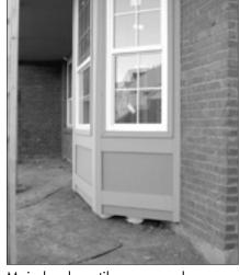
Main level cantilevers posed access challenges because they were so close to grade. There was no soffit on this one. The construction superintendent was aware of the problem and planned to dig a hole
