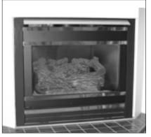
Three types of natural gas fireplaces were observed in study homes: atmospheric gas log sets with operable glass doors (left), atmospheric fireplaces with solid glass facades (center), and direct-vent units (right). The atmospheric units rely largely on house air for combustion and dilution air, whereas the direct-vent units draw all required air directly from outdoors.
