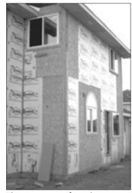
The coverage of insulating foam sheathing on study homes ranged from zero to 100%. When it was present, coverage averaged about 60%. The typical foam sheathing was nominal 1/2-inch extruded polystyrene, rated at R-3.
