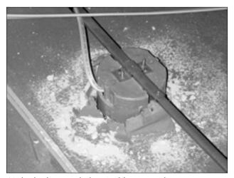
Air leaked around electrical boxes and through wiring penetrations.
