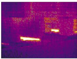
Uninsulated. Strips of concrete exposed above grade in this stepped foundation stood out as hot spots compared with the insulated frame wall and earth. Eight inches of concrete provide only about R-1 resistance to heat flow.
