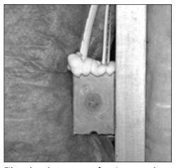
Fiberglass batts were often improperly fit around obstructions like this electrical box, creating cold spots. (This is the back of the box; code requires a minimum of R-5 insulation behind such obstructions.)
