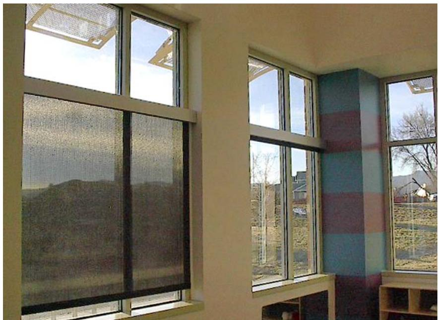
*South-facing windows are shaded by perforated roller shades and perforated overhangs.*
