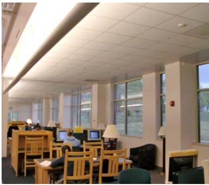
Adjustable indirect luminaires provide general lighting along the periphery.
