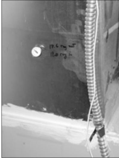
The only way to know whether a furnace is operating within the manufacturer-specified heat rise range is to measure heat rise. This test requires minimal tools and time. The testing contractor saw no evidence that heat rise had been measured on study home furnaces.
