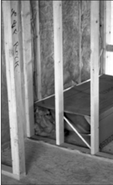
This bathtub had more than enough insulation at the exterior wall. But there was no air barrier to stop air from the outside wall from flowing through the insulation and circulating beneath the tub. From there, connections through partition walls and holes around the plumbing connected this leak to the rest of the house.
