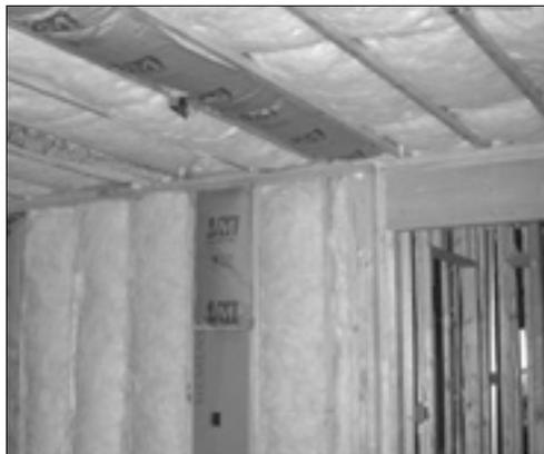
In floors over garages, R-30 batts exceeded code R-value requirements but were easier to install effectively because they were thick enough to fill the floor joist cavity completely.
