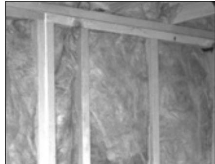
Typically-installed, unfaced fiberglass batts in a frame wall will offer reasonable performance. Note some compression of the batts in the full-width stud bays and more severe problems where a batt had to be cut to fit in a narrow cavity.
