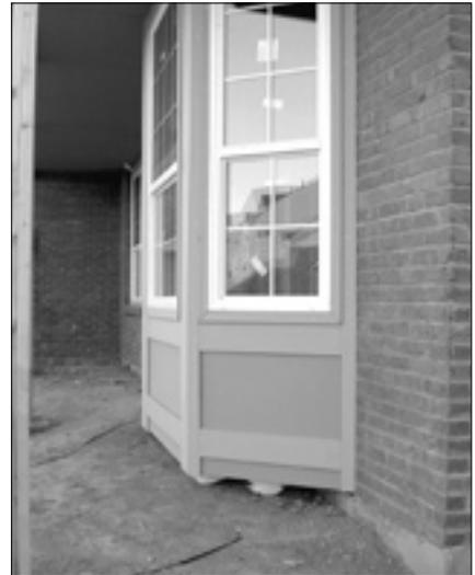
Main level cantilevers posed access challenges because they were so close to grade. There was no soffit on this one. The construction superintendent was aware of the problem and planned to dig a hole to be able to install it.
