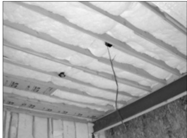
Code requires minimum R-19 insulation in floors above garages. The insulation must be in substantial contact with the subfloor above, permanently supported using one of several approved means. In this example, 6-inch thick R-19 fiberglass batts, installed in 9.25-inch joist cavities, were held in place only with staples—not an approved method. Some of the staples had failed prior to wallboard installation.
