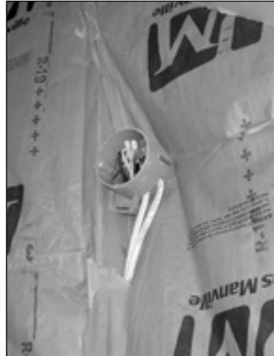
The code requires that insulation be cut to fit, without compression, around electrical and other obstructions in the insulated bay. In this case, insulation was compressed behind the box rather than cut to fit around it.
