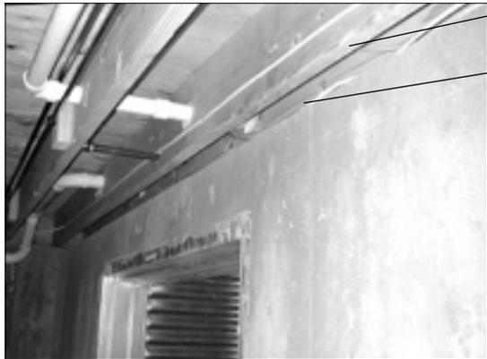
When the first floor joist was framed tight to the foundation, it left little space to insulate the rim joist. Plumbing and wiring complicated the job in this example.
