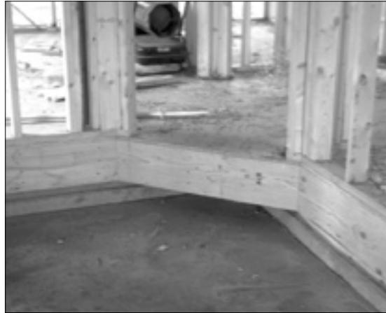
Many holes were observed between garages and houses, providing pathways for garage pollutants to move into the living spaces. This corner cantilever was liable to be a big leak because it was difficult to access to seal.
