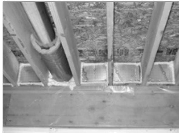
This photo illustrates an effective sealing job. Easily cut material, sealed at the edges, blocks air movement through the cantilever.
