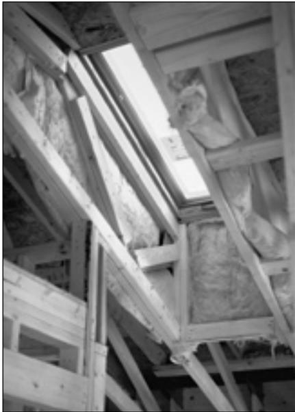
The code requires insulation to be in substantial contact with the wallboard and a vapor barrier to be installed on the warm side of the insulation. At this skylight well, insulation was held several inches back from the wallboard by framing. The vapor barrier was on the cold side of the insulation, a potential moisture trap.
