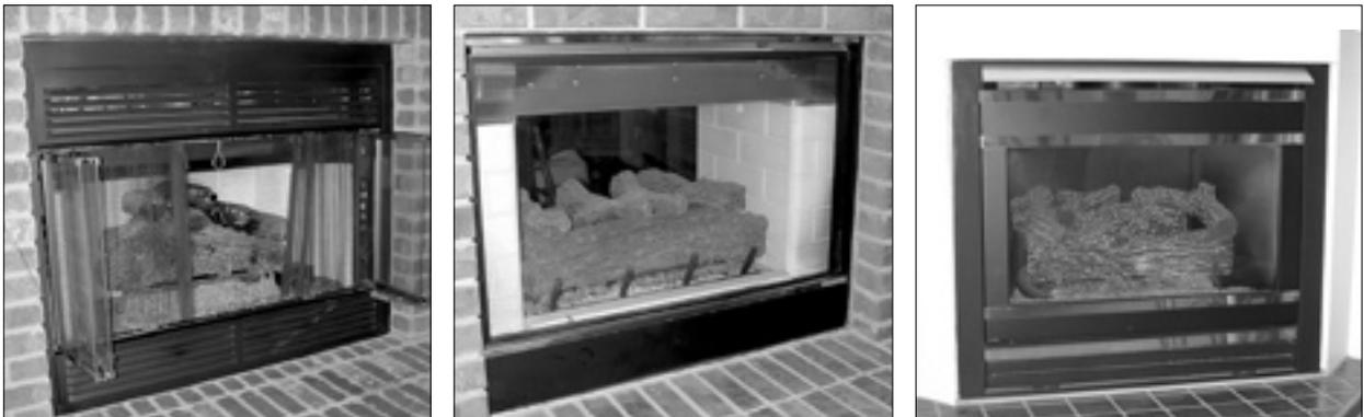
Three types of natural gas fireplaces were observed in study homes: atmospheric gas log sets with operable glass doors (left), atmospheric fireplaces with solid glass facades (center), and direct-vent units (right). The atmospheric units rely largely on house air for combustion and dilution air, whereas the direct-vent units draw all required air directly from outdoors.
