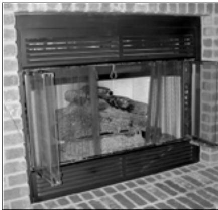
The flue, draft hood and outdoor air supply all contributed to leakage through atmospherically vented fireplaces.
