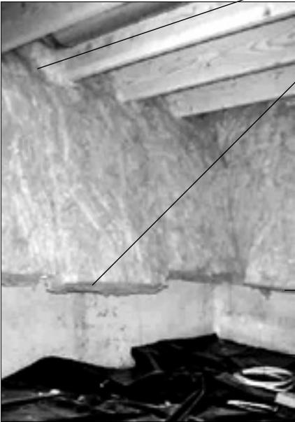
Insulation was compressed where it attached to the rim joist.
