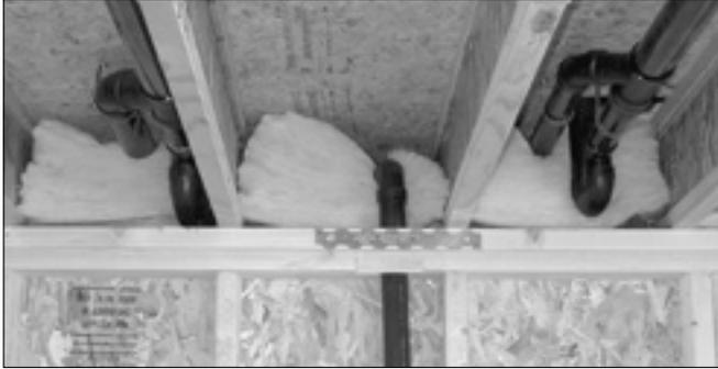
Compression of the insulation batts, voids, and the lack of contact with the subfloor above this cantilever all reduce the effective R-value of this insulation.
