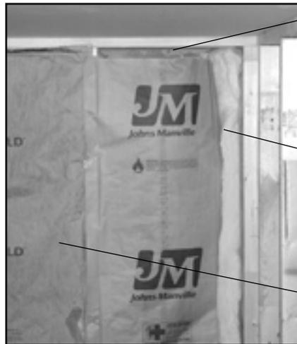
One-inch void at top of wall cavity
