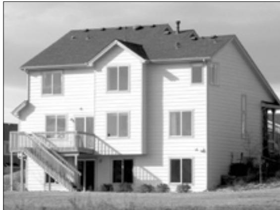
Some study homes had a lot of south-facing glass area, offering the potential for great passive solar performance. However none were designed to take advantage of the solar heat during the winter (by storing the heat) or to avoid the sun during the summer (with exterior shading). During the winter, these homes tended to have large temperature variations from one part of the house to another.
