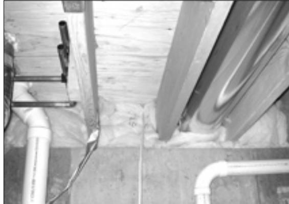
Many obstructions—such as the plumbing and ductwork shown here—made it harder to insulate rim joists effectively. Even where nothing was in the way, insulation was sometimes placed in cavities with insufficient attention to detail. Also note there was no vapor barrier to prevent moisture from reaching the rim joist.
