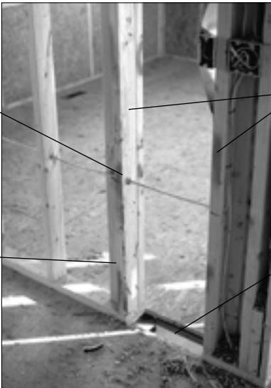
These wall studs formed two sides of a return duct. Wallboard will complete the other two sides.
