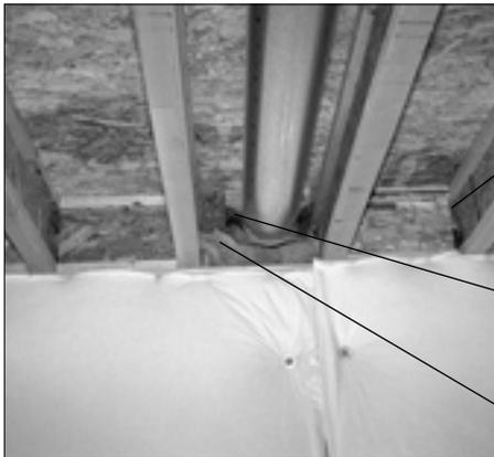
Rectangular blocking coupled with engineered "I-beam" joists left large gaps at the edges.
