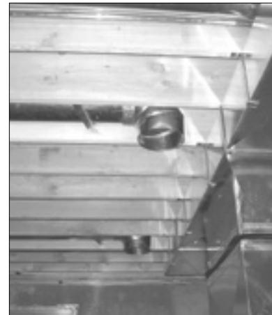
To help maintain a safe combustion environment, code requires large combustion air openings in the vicinity of atmospherically coupled combustion appliances. Testing showed that these ducts had very small beneficial effects on basement depressurization. In fact, when the wind blows in certain directions or when the exterior end terminates in an attic, ducts like these can drive the basement pressure more negative.
