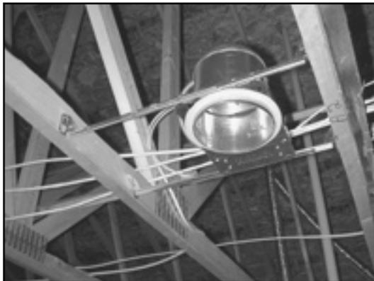
“Airtight” cans for recessed lighting reduced air leakage through insulated ceilings.
