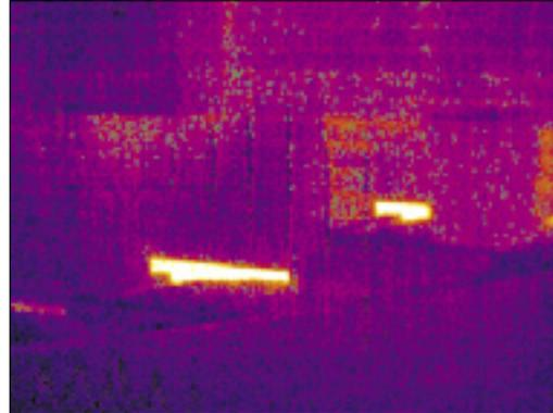
Uninsulated. Strips of concrete exposed above grade in this stepped foundation stood out as hot spots compared with the insulated frame wall and earth. Eight inches of concrete provide only about R-1 resistance to heat flow.
