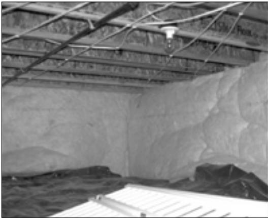
In this crawl space, insulation was effectively installed. This should ensure that the rated R-value will be delivered.
