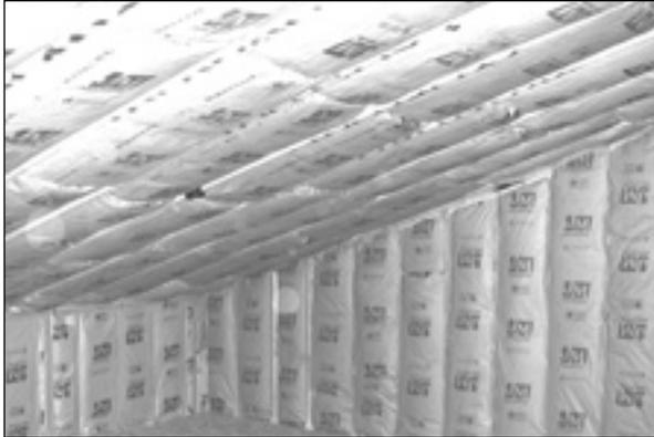
This is an example of effectively installed insulation that met code requirements. Batts filled the cavities, attained full loft, and will be in substantial contact with the wallboard.
