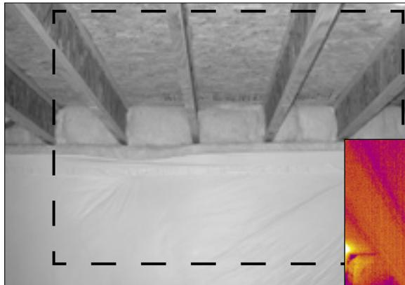
The infrared photo (right) shows the symptoms of compressed insulation and air leakage at the rim joist.
