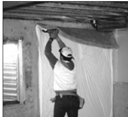
Basement wall insulation addressed one of the biggest remaining heat loss paths. The typical approach was a vinyl-faced fiberglass blanket on the interior of the concrete foundation.
