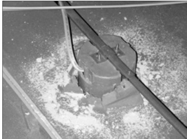
Air leaked around electrical boxes and through wiring penetrations.
